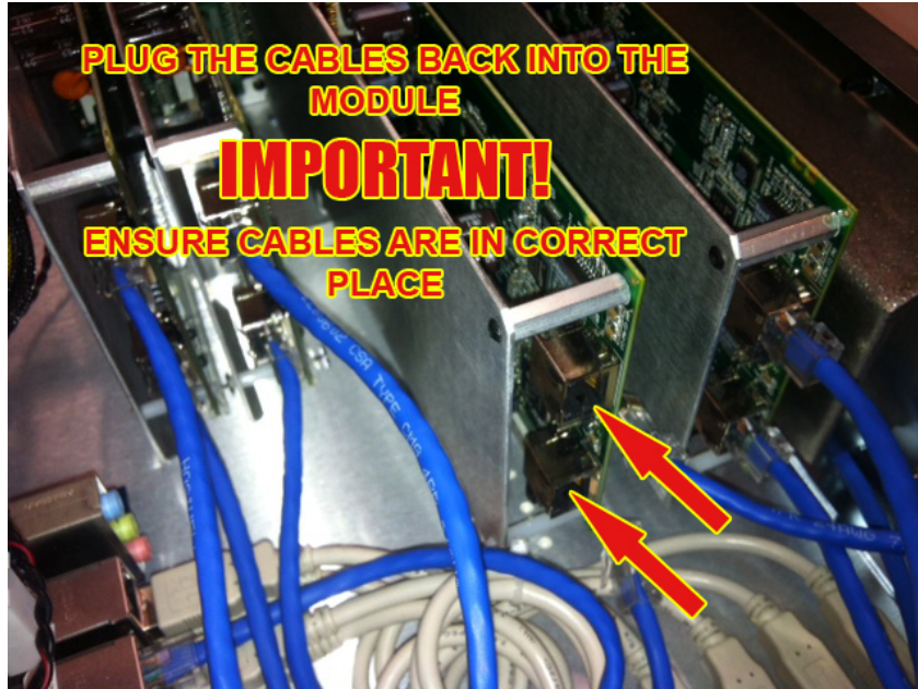
Figure 13-8 Plugging Cables into the New Control Module
