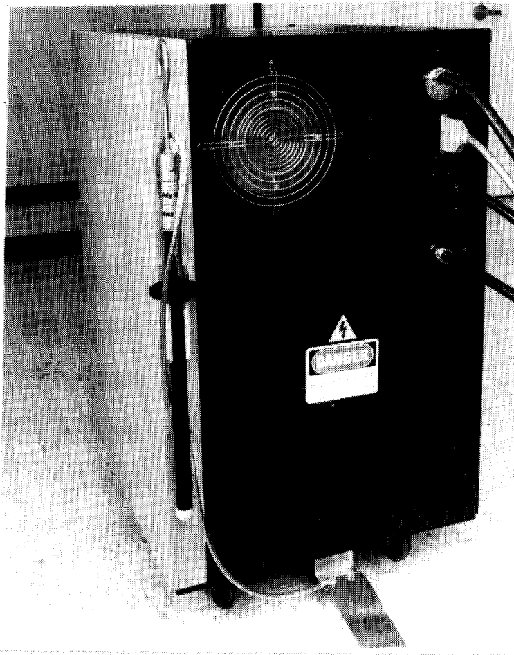
Figure 2-9. Rear of Power Module, with Grounding Hook and Low-Impedance Copper Ground Strap Correctly Installed
